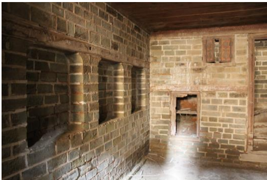
Fig. 30 View of the basement
