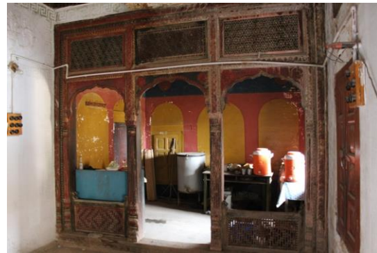
Fig. 20. Room with wooden partition
