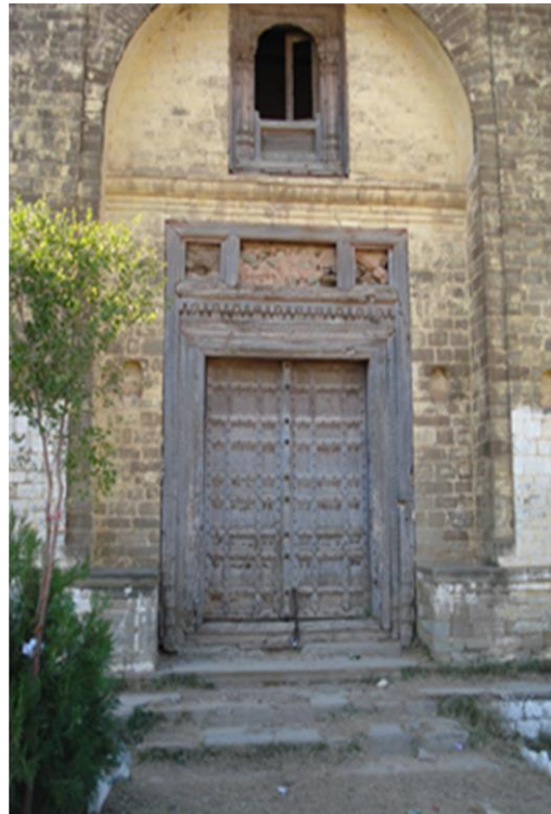
Fig. 9. First entrance door
