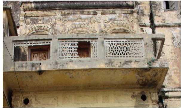
Fig. 24. Balcony from first courtyard
