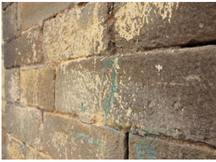
Fig. 7. Stone bricked wall
