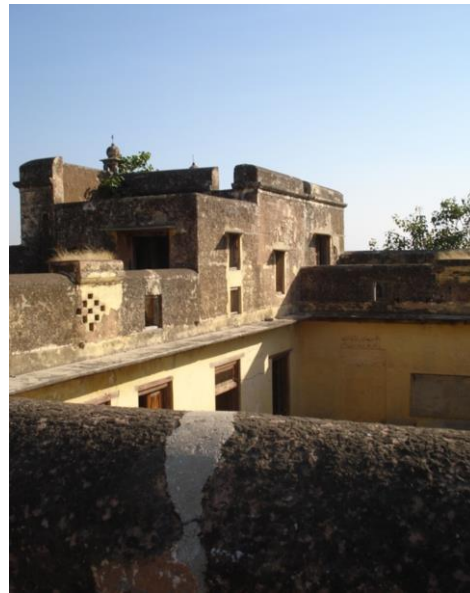
Fig. 28. View of guard room and parapet wall
